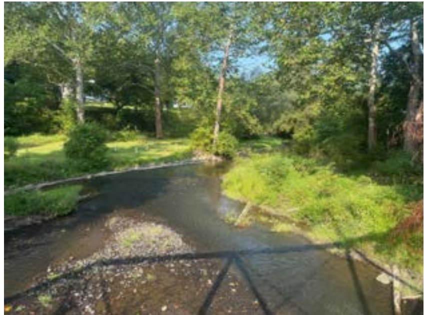
Woodcock Creek at Craig Road Post Restoration. The single-log vane deflectors are on the right of the image, and the mud sill cribbing on the far part of the stream
