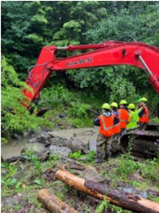
Our summer WCRC technicians assist with the contractors installing new support structures at German Run at Telliho Property During Restoration - June 2023
