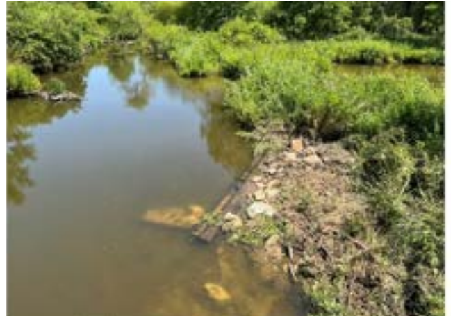
Log Framed Stone Deflector
