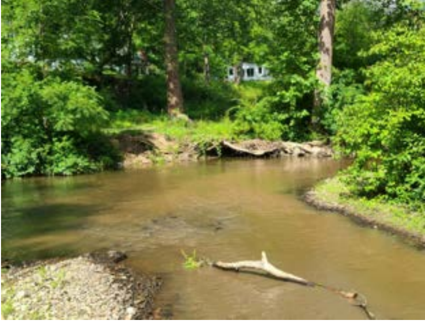
Woodcock Creek at Craig Road Pre Restoration - July 2022. Notice the undercut banks on the far side of the image
