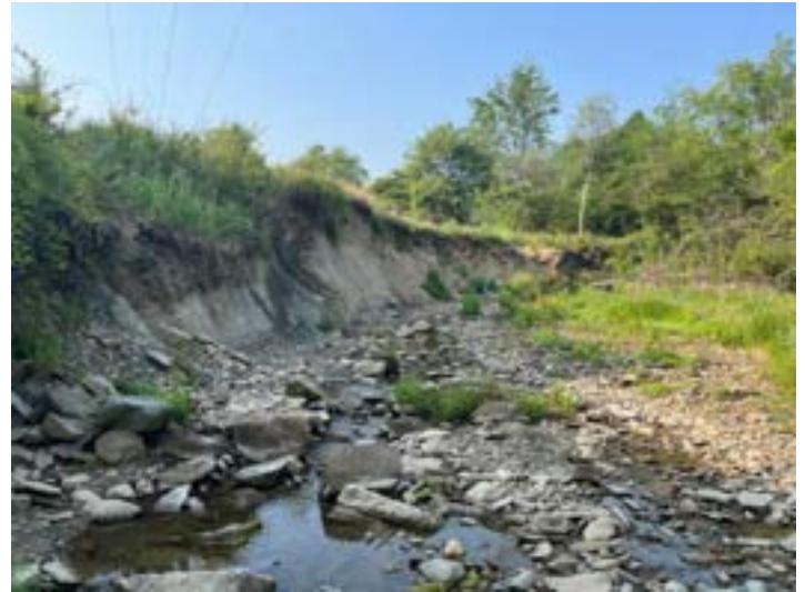
German Run at Telliho Property. Notice how much of the bank has been washed downstream. Pre Restoration - May 2023
