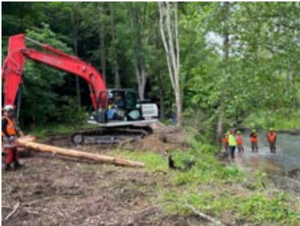
Woodcock Creek at Stainbrook During Restoration - June 2024
