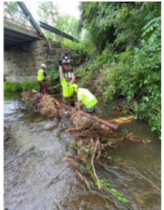
Root Wad Deflector during installation
