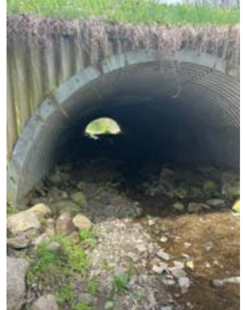
Recently Replaced Cylindrical Culvert at Stream Grade
