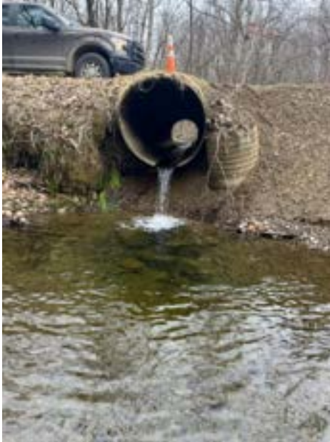
Traditional Circular Culvert Design with Head Drop
