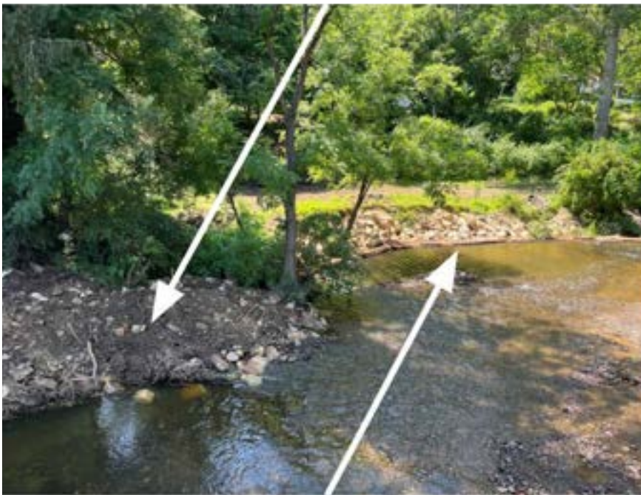
Mud Sill Cribbing
