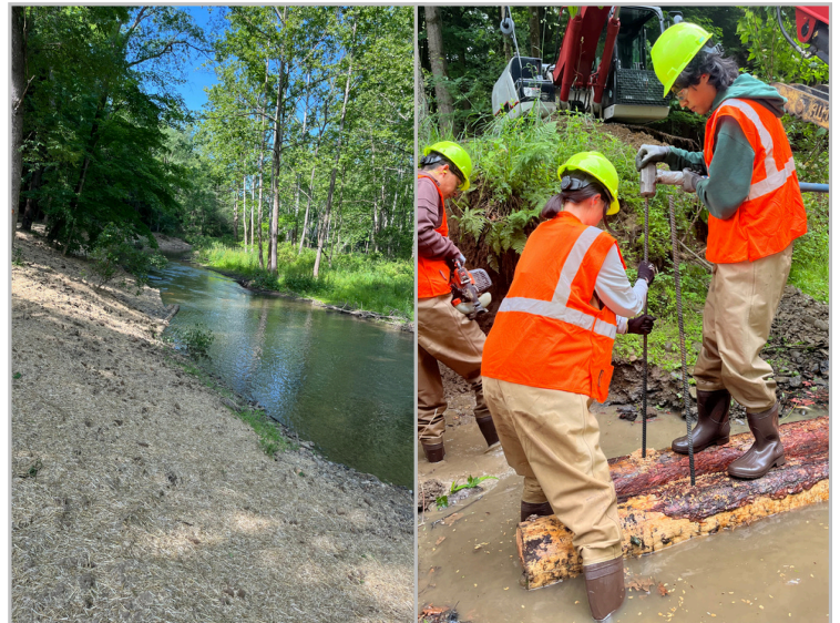
Left: Instream habitat improvement during the last phase of construction
