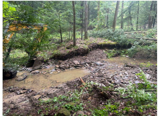
Added wood increases in-stream habitat diversity
