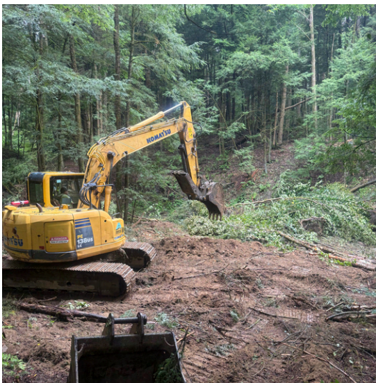
Excavator used to position felled trees within stream
